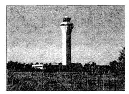
The MCI ATCT has experienced significant past water incursion problems, as well as interior moisture issues that have led to mold growth and resulting remedial efforts. Reports reviewed as part of the inspection process indicate that mold remediation work was completed within the MCI tower in 2003 and 2007, and that the exterior caulking on the tower shaft was replaced in the 2004/2005 time frame. The original caulk reportedly degraded over time as a result of ultraviolet light exposure.
